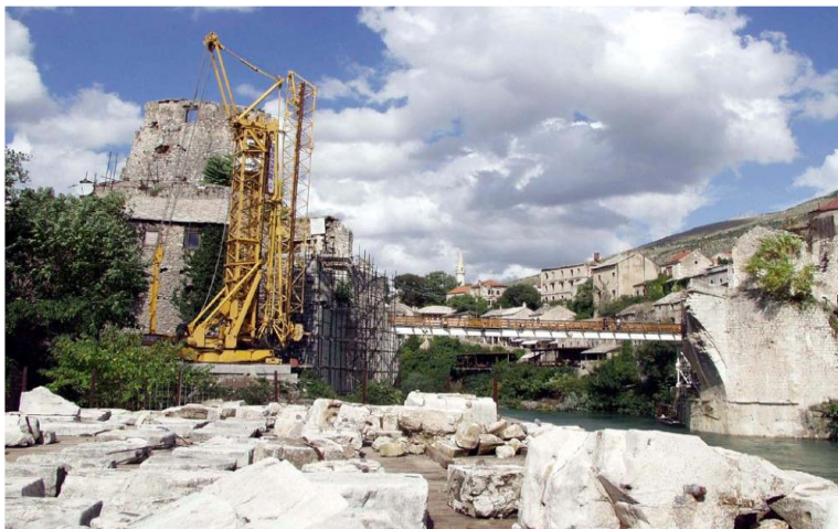
Picture 8: The start of reconstruction of the Old Bridge, mounting of the first crane and scattered stone blocks on the platform by the river
