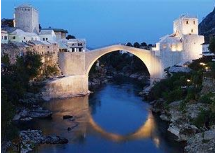
Picture 17: A “new” Old Bridge
