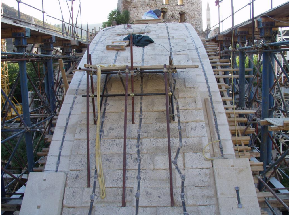
Picture 16: A view on finished arch (east side)
