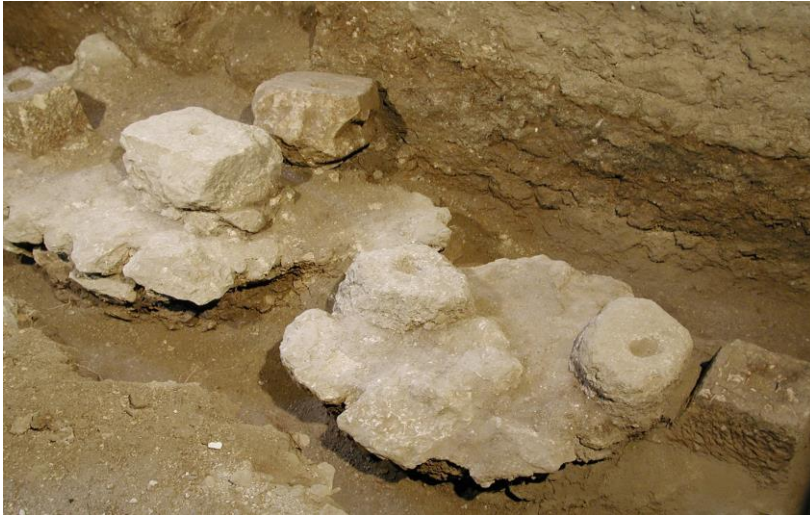
Picture 5: Stone foundations of one path which led to the medieval wooden bridge (they were found underground and they contain openings for placement of the wooden consoles)
