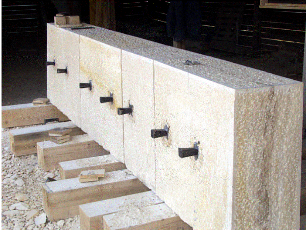
Picture 13: A row of four stone blocks prepared for mounting
